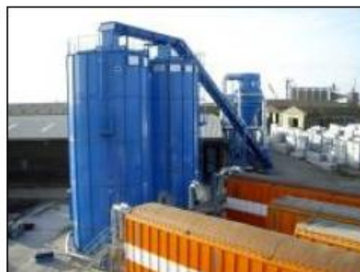
Silo and conveyor
