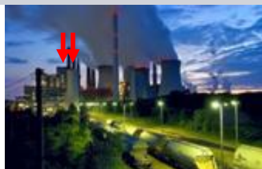
Neurath D&E, Niemcy 2 x 630 MW, Lignite → Tangentially Fired → Increase of Efficiency → Reduction of Slagging → Expand Control Range
