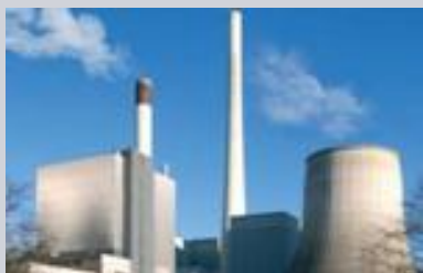
Elverlingsen, Niemcy 1 x 330 MW, Hard Coal Melting Chamber Furnace → Increase of Biomass Co-Combustion
