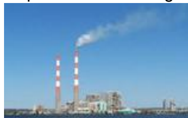
La Cygne 2, USA 1 x 710 MW, Hard Coal → Opposed Fired → NO x -Reduction
