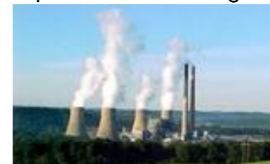
Keystone 4, USA 1 x 936 MW, Hard Coal → Opposed Fired → Increase of Efficiency
