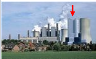
Niederaußem K, Niemcy 1 x 1000 MW, Lignite → Tangentially Fired → Increase of Efficiency → Reduction of Slagging → Expand Control Range
