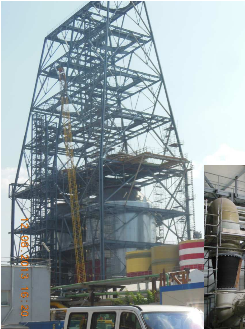
2 Absorbers with steel structure for the stacks
