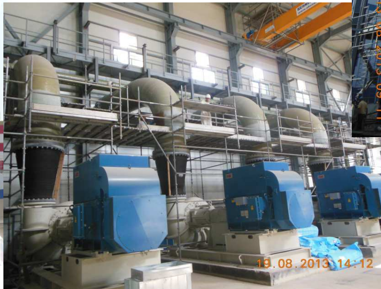
Absorber recycle pumps
