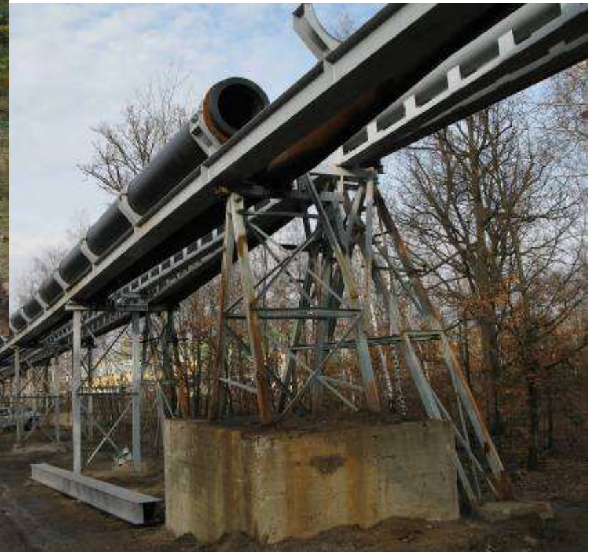
WehoPipe DN 900 SDR 17 L=1650 m
