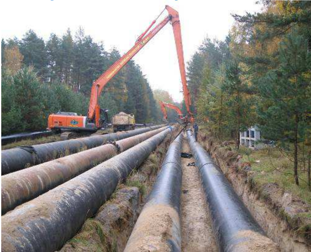
WehoPipe DN 1000 SDR 11 L=4950 m
